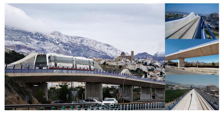
The Altea railway viaduct was designed and constructed with a ribbed deck, which presents the singularity of a central web designed to increase depth above the deck. The superstructures' main features are:
